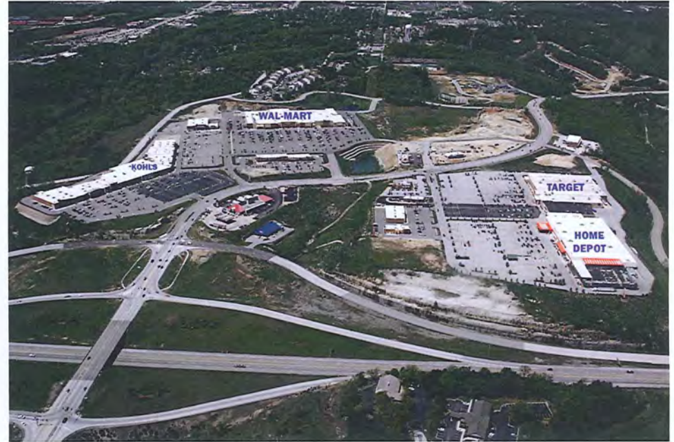
Aerial View Looking West
